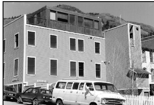
As seen from the rear, the third floor appears as a subordinate additive form (see above photo).
