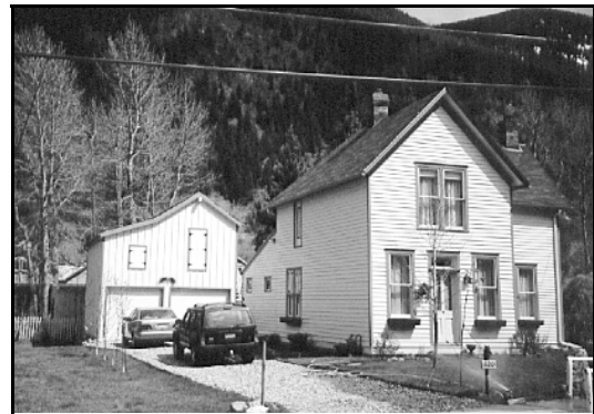
Preserve an historic structure in its original location on the site.
