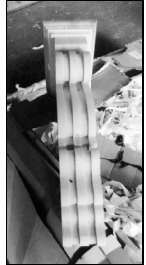
Replacement of missing architectural elements should be based on accurate duplications of original features.
