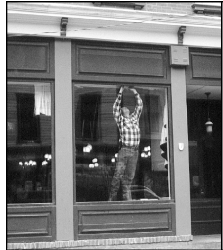
Employ treatments such as rust removal, caulking, limited paint removal and reapplication of paint.
