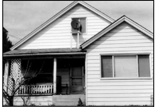
A small satellite dish should be mounted in the least visible location possible.
