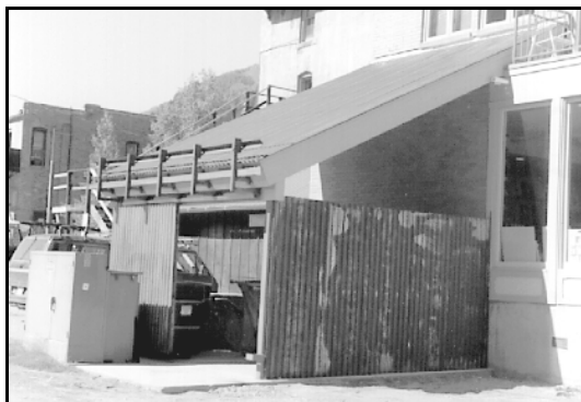
Trash areas for commercial uses should be screened from view, using a fence, hedge or enclosure.
