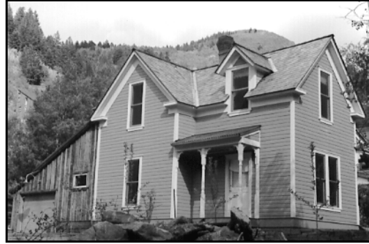
A substantial addition should be distinguishable from the historic building so it can be understood as a more recent change. This can be accomplished with a subtle change in material.
