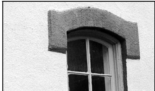
Where a covering of stucco has taken on historic significance, consider repairing damaged areas and periodic cleaning.
