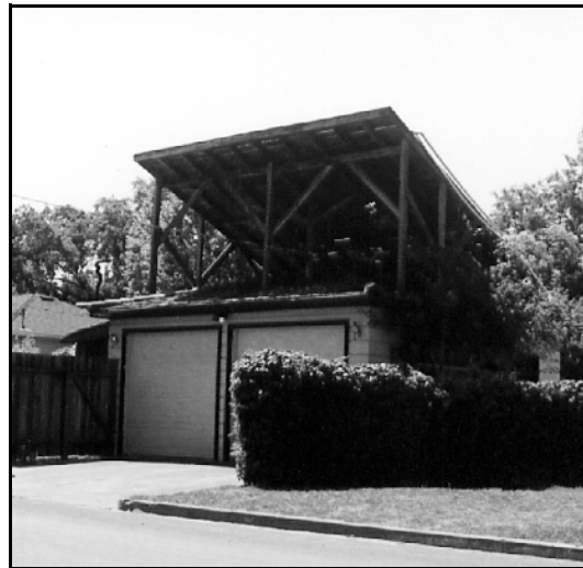
If attached to the building, solar devices should lay flush with the roof line. This device is inappropriate.
