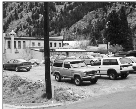
Minimize the visual impact that large areas of parking create. This lot is not screened or landscaped and is discouraged.
