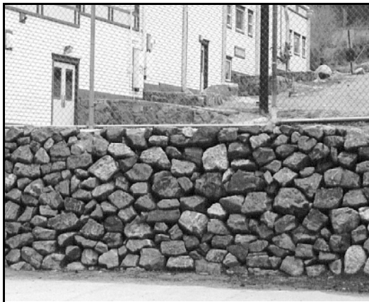
For a replacement retaining wall, use materials that appear similar to that of the original.
