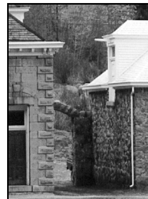
Some of the more prominent buildings in the residential areas were constructed of masonry.
