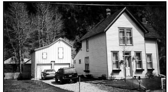
Additions and accessory structures should be set back from the front of the primary structure.
