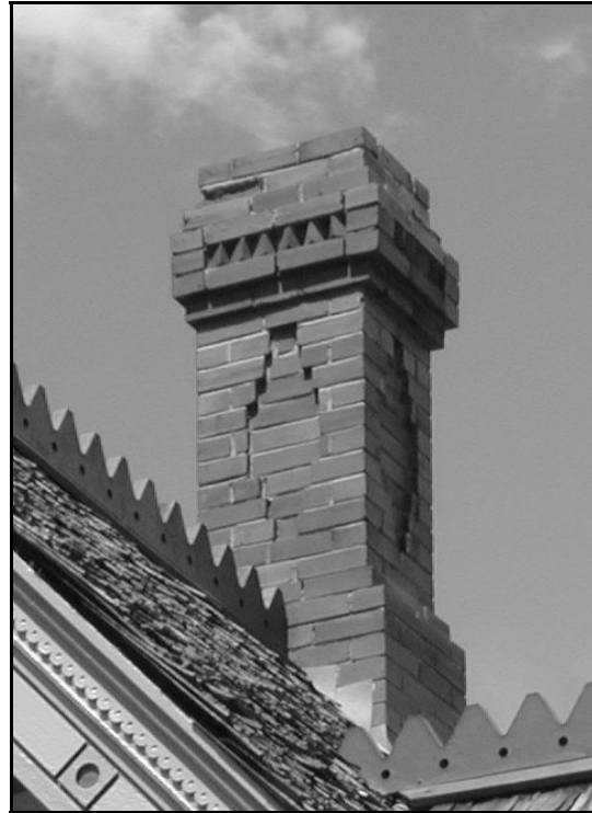
An historic chimney should not be removed.
