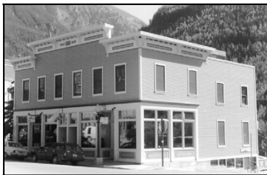
This new storefront is clad in wood siding and uses traditional historic details quite accurately. A stepped cornice expresses the traditional façade widths of the street and upper story windows have traditional trim.
