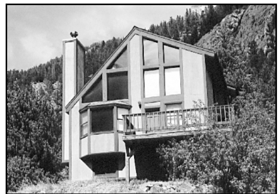
Large areas of glass in exterior walls that may allow "spill-over" of interior light sources, resulting in nighttime glare, should be used with caution.
