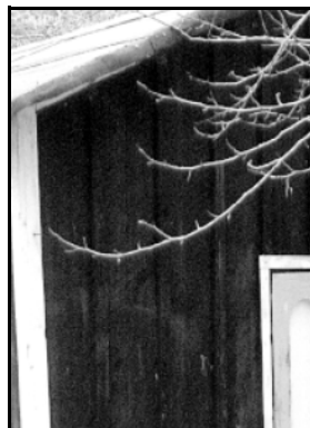
Board and batten siding was a common building material for secondary structures.
