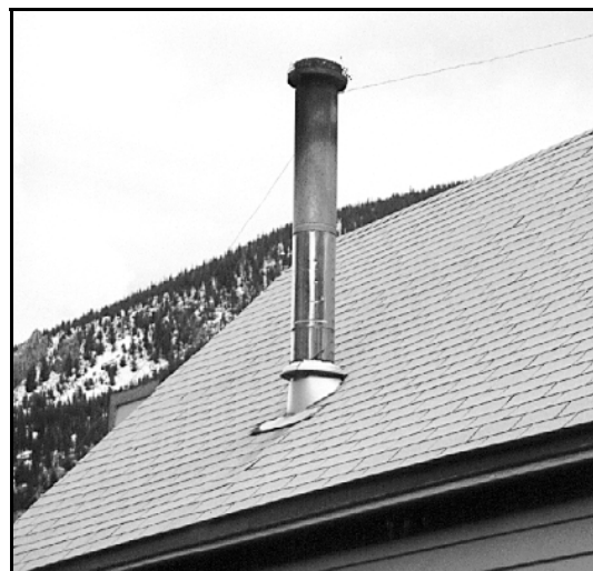
A stovepipe, on any building, should have a matte, non-metallic, dark finish. The bottom half of this stovepipe is reflective and is inappropriate.
