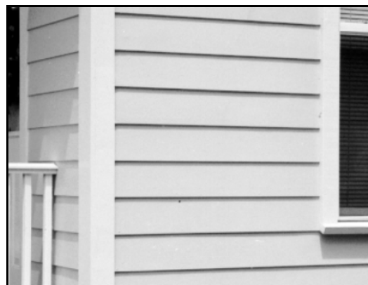
Synthetic materials, such as this composite cement board, may be considered if they appear similar in character and detailing to traditional building materials.
