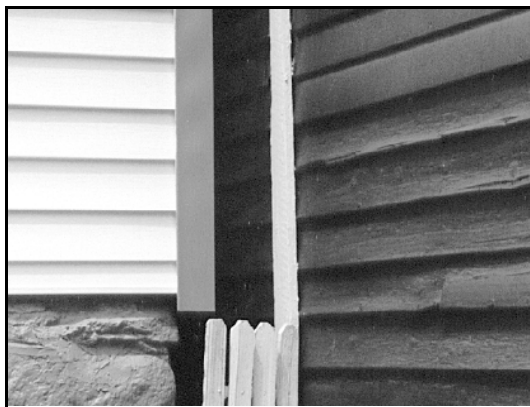
Protect wood features from deterioration. If the building was painted historically, it should remain painted, including all trim.
