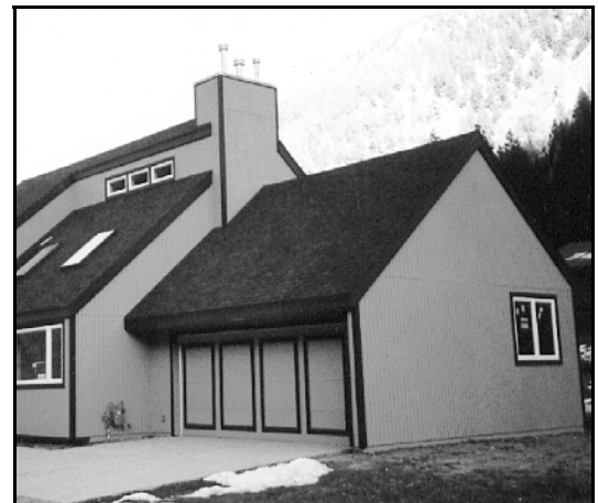
In new construction, a clear distinction between foundation and wall material should be present. For example, wood siding should not extend to the ground.
