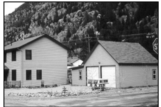
Construct an accessory structure that is subordinate in size and character with the primary structure. This one is too big compared with the primary structure, and is inappropriate.
