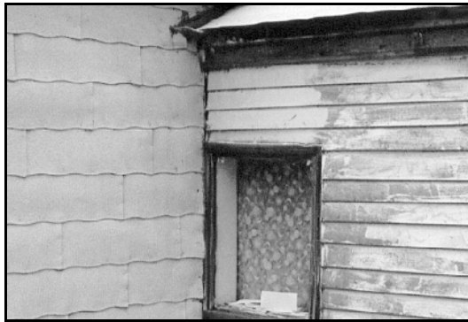
Original building materials should not be covered. If original materials are presently covered, consider exposing them;
